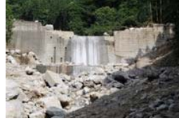
梨子沢砂防堰堤
